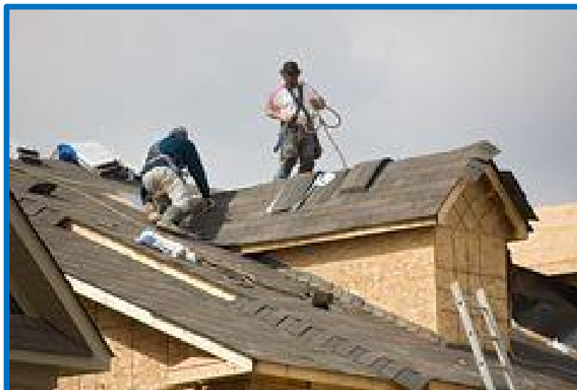
Workers replace a roof at a CHI project.
